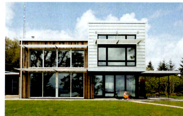
The mix of materials gives the home’s exterior a textured look. The salvaged barn wood highlights the living area, and the corrugated metal highlights the bedrooms.
